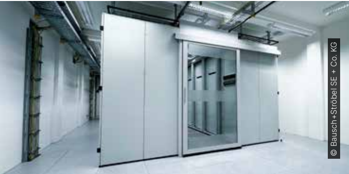
View into the server room of the outdoor data center with cold and hot aisle containment
